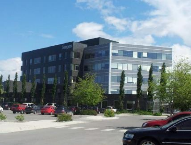
Centerpoint Financial Center Anchorage, Alaska
